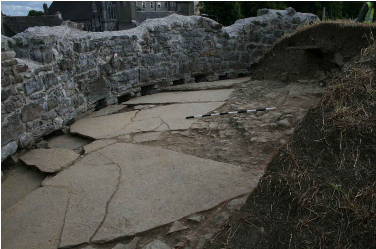
Flagstones on the southern perimeter of the roof
